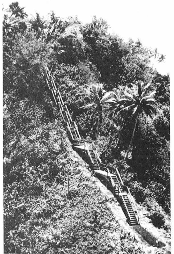
Figure 9. Access stairway from Lauagae Ridge to Matatula Point.
