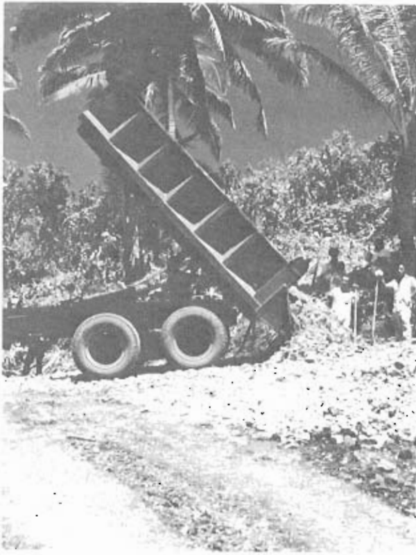
Figure 3. Initial road construction, Samoa.
