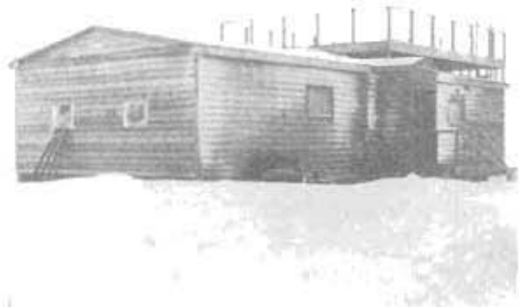
Figure 9. Completed Barrow Observatory, October 1972.
