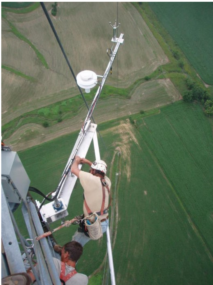
Figure 1. Air Intake at West Branch Iowa Tower.
