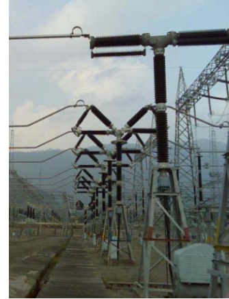
400 kV SF 6 Circuit Breaker
