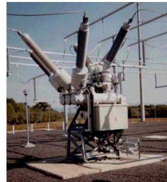
Hybrid Switchgear
