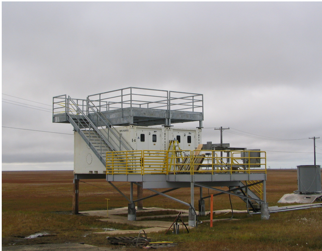
Figure 1. Additions to an existing deck near the main ARM Barrow instrument shelter, 9/05. Side by side shelters with deck above for upward-looking instrumentation. Addition doubles shelter space for instrumentation at the ARM Climate Research Facility, Barrow, which is adjacent to the NOAA GMD Barrow Station.
