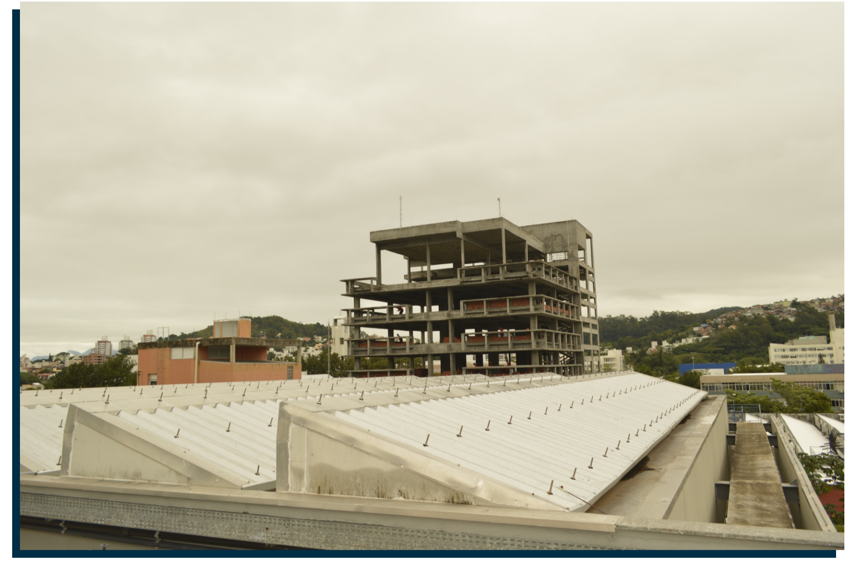
View of the eight floors laboratory building from the roof of the solar energy laboratory building.
